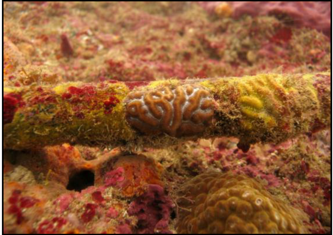
Telecommunications cable with encrusting marine organisms
