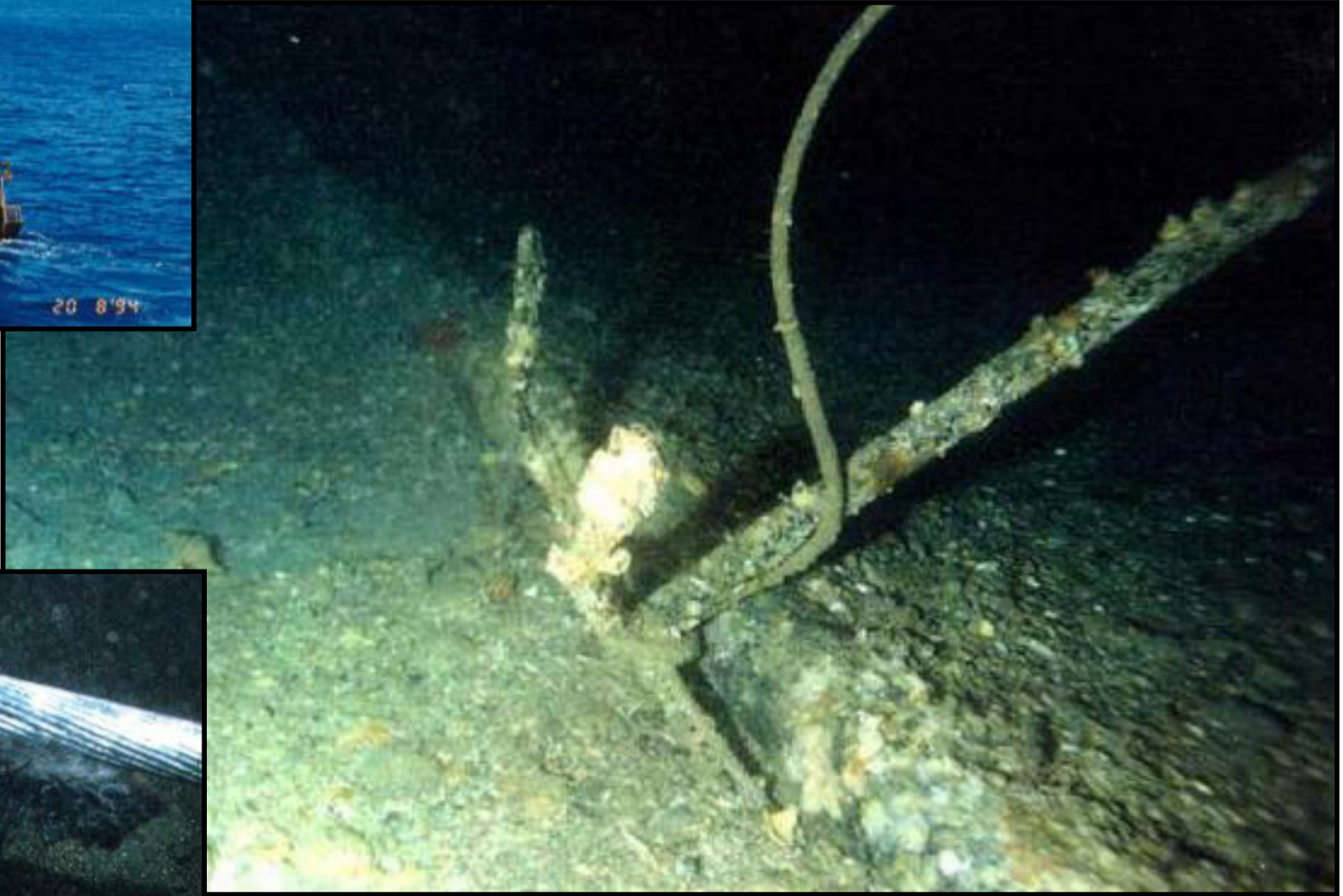
Cable snagged and moved by trawl gear
