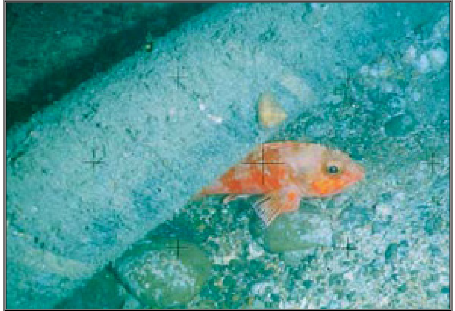
126mm diameter power cable in Submarine Cable Protection Zone across Cook Strait, NZ
