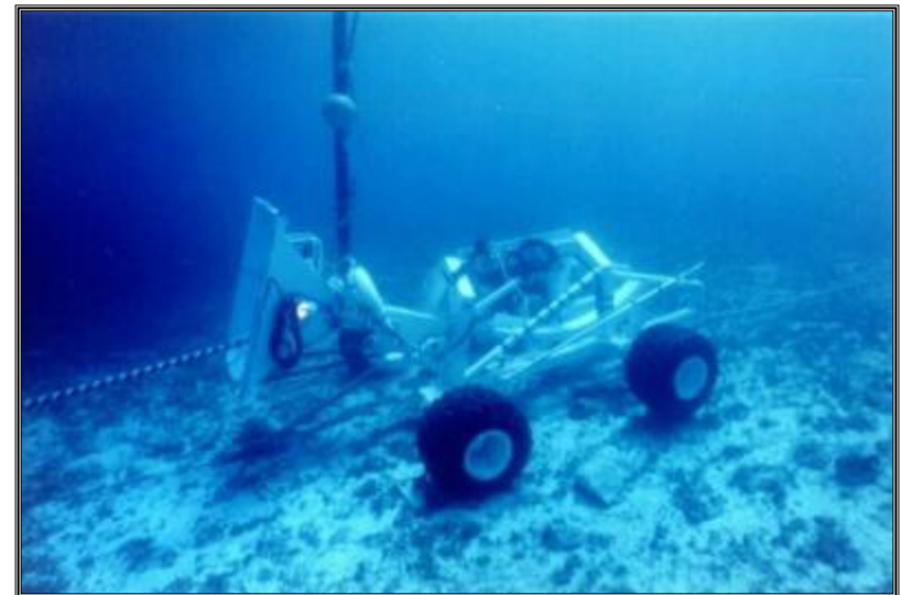
Power cable installation using Hydroplow
