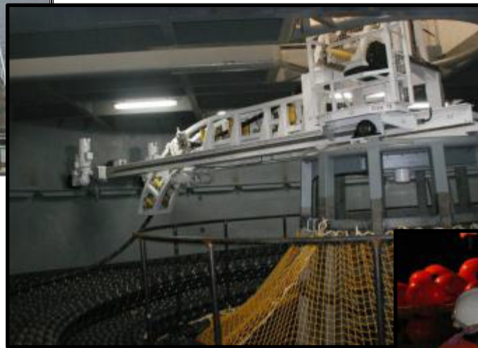
Loading/unloading arm in cable storage tank
