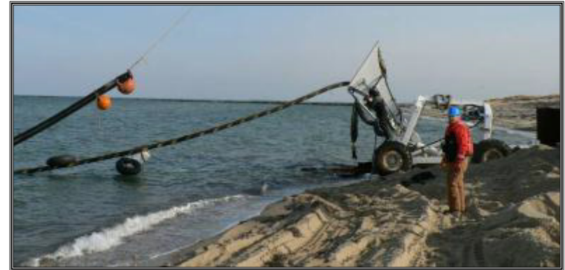
Power cable installation using Hydroplow
