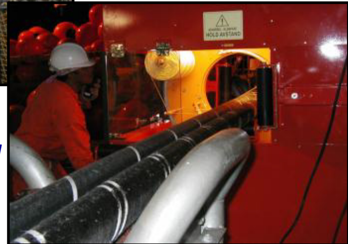
“Bundling” power cables for laying
