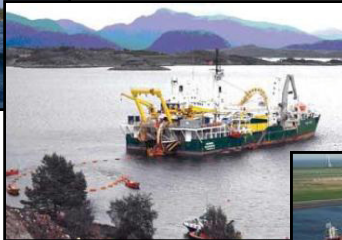
CS Skagerrak installing 420 kV Cable
