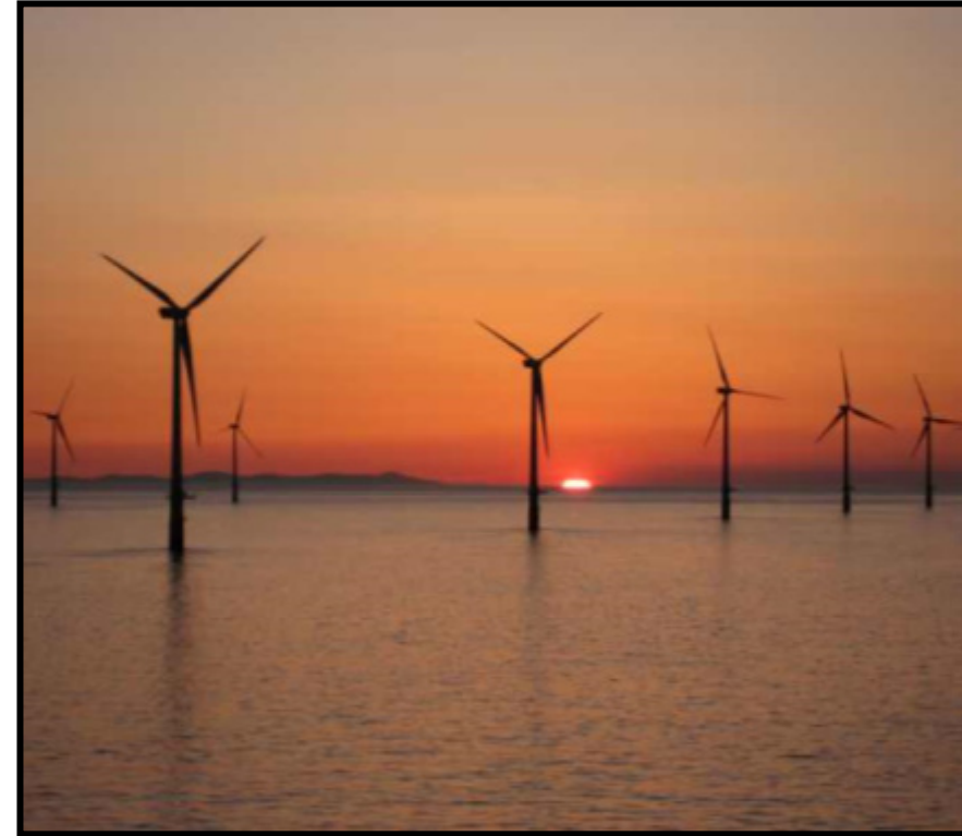
Offshore wind farm
