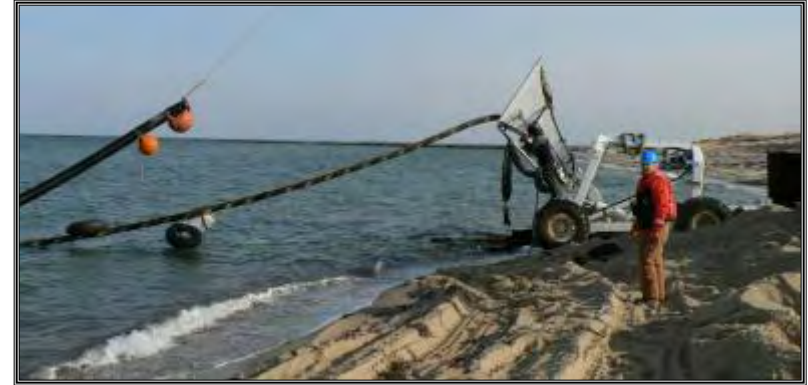
Power cable installation using Hydroplow
