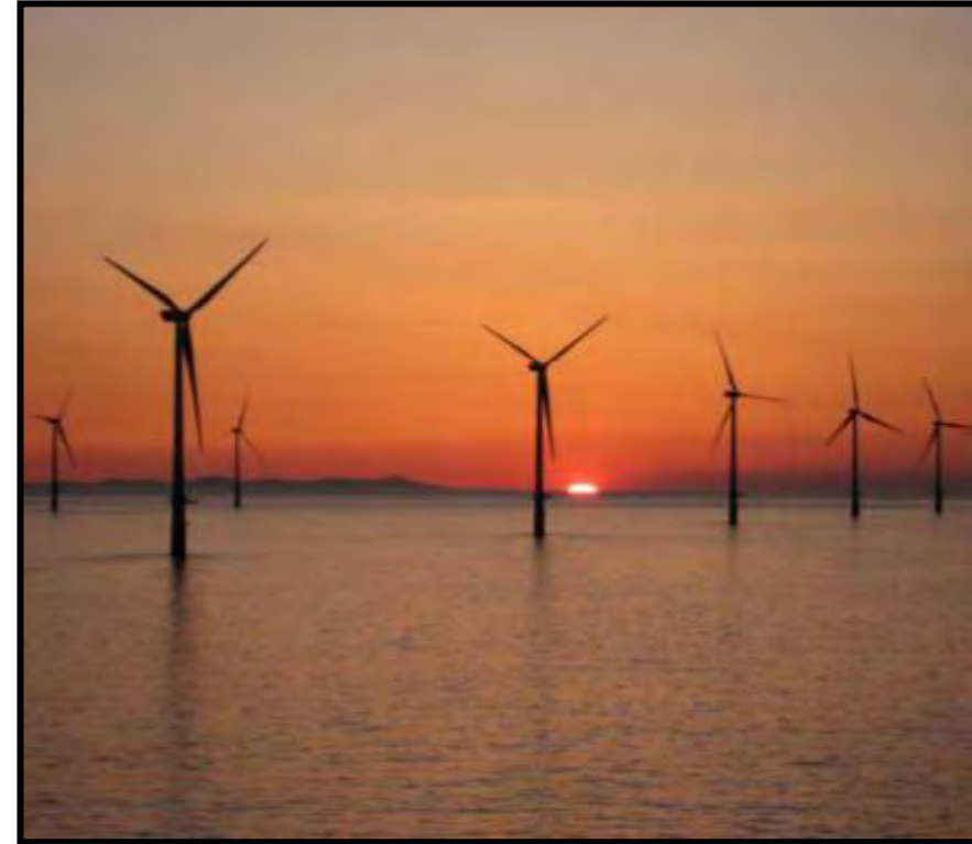
Offshore wind farm
