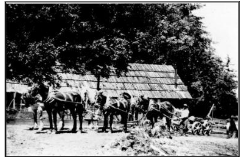
Horses pulling submarine power cable ashore to form terminal, around 1930; Washington, USA
