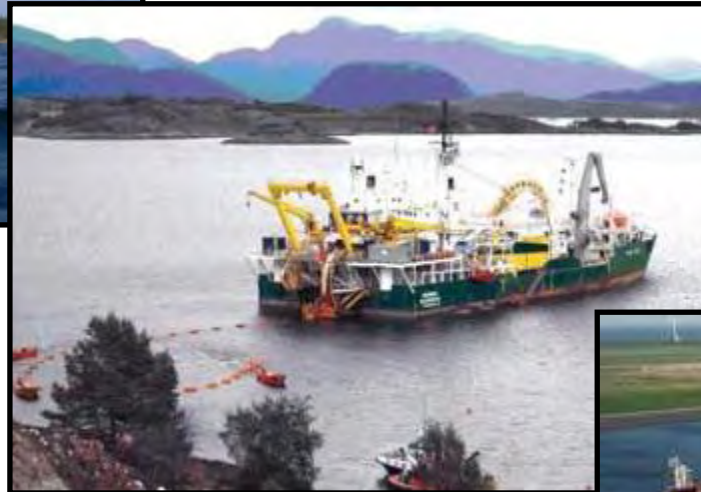
CS Skagerrak installing 420 kV Cable
