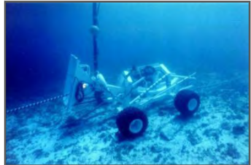
Power cable installation using Hydroplow
