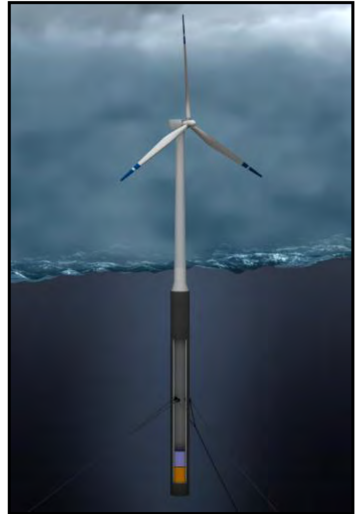
Hywind floating wind turbine can be moored in water depths up to 700m
