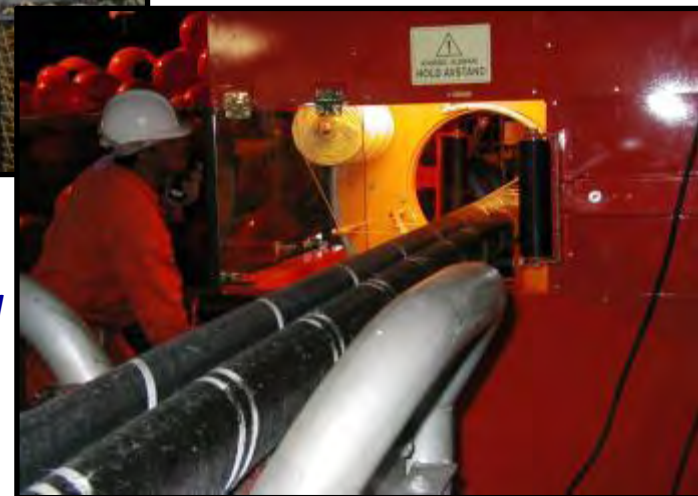
“Bundling” power cables for laying
